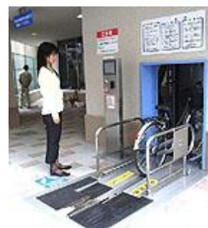
3. The gate opens and the bicycle is stored automatically.
